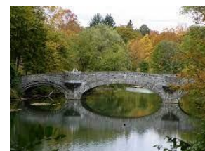
The elegant stone footbridge over the Susquehanna in Cooperstown frames the start of the May 14th paddle.
